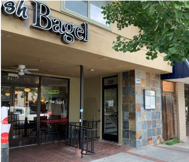
West façade, stairwell, ESA 2022
